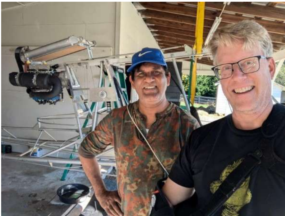
Arvind Singh and Shawn Lillemo have the engine, muffler, and radiator installed
