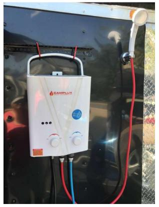
The tankless heater mounts outside the trailer because it also acts as an outdoor shower (yes I have a stand up tent) and the hoses have quick connectors that run under the trailer and inside to the sink. And with a tankless water heater you have to have propane on board so figured I might as well get one of those propane fire pits so we don't always have to gather wood and smell like smoke. That setup lasted a few months until I thought of more.
