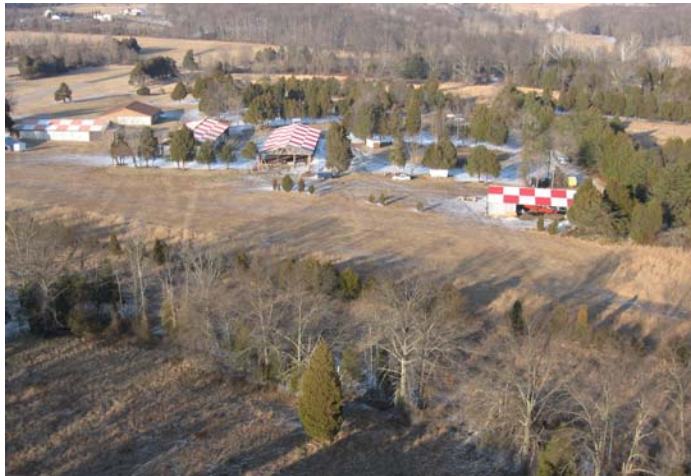
New Hangar Roof
